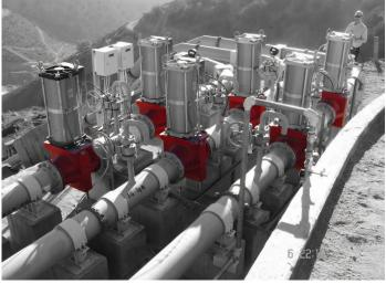
construction of the Flowrox valve ensures that the valve closes tightly even if coarse particles remain between the closing device. In the open position, the valve is actually a part of the pipeline. In some cases,
