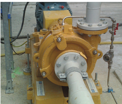
Fig 2: Heavy duty slurry pump type Ensival Moret EMW with high abrasion and corrosion resistance
