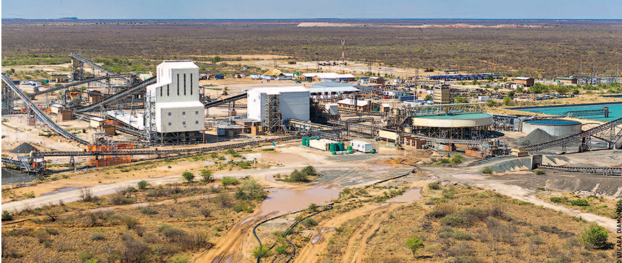
Lucara's Karowe mine in the Orapa kimberlite field of Botswana. The tall building in the centre houses the TOMRA XRT sorters.
